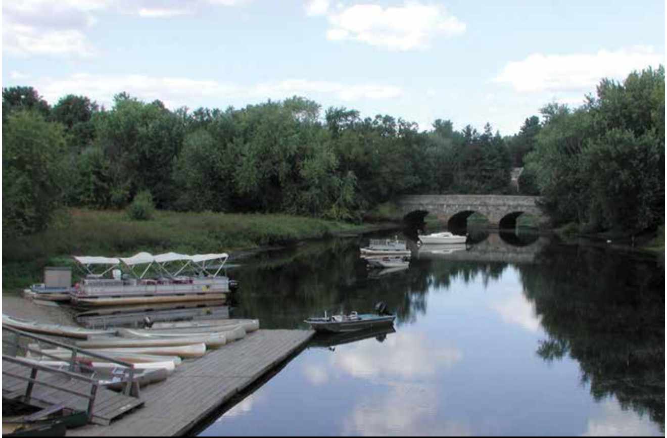
The Council has been involved in numerous projects to help preserve and enhance the historic and scenic bridges in the region. PHOTO COURTESY OF OARS
