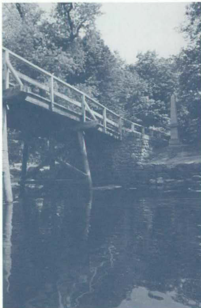
North Bridge, Concord.
